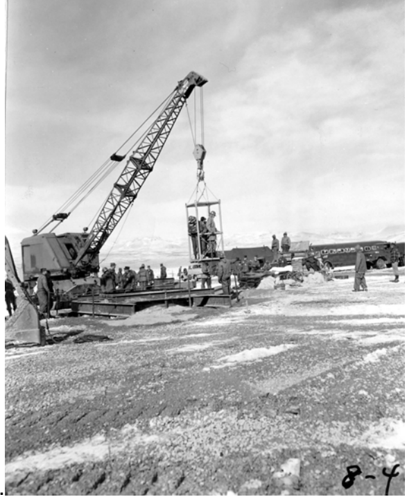
PLK 8-4 - 19Jan55 "Bird Cage" going down ESS shaft
